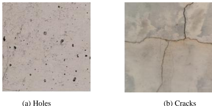
Figure 1. Apparent defects in fair-faced concrete
