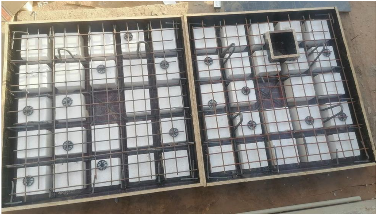
Fig.2 Waffle formwork
