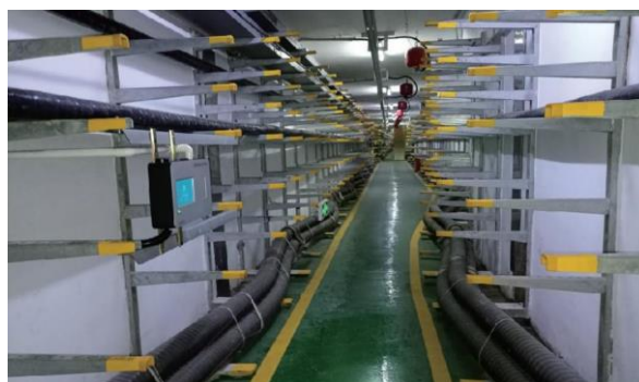
Figure 6. Multi-level fire alarm system installed in high-voltage tunnel
